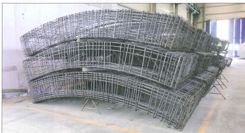
Above: Steel cage bars for the segments had to be reduced in diameter to increase reinforcement
