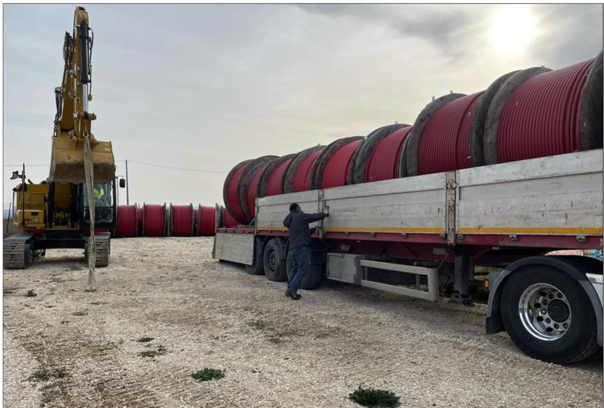
Figure 11-8 - MV cable unloading at site
