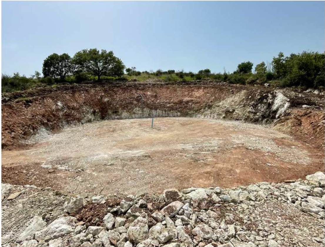
Figure 11-2 - Works on site for WTG 18
