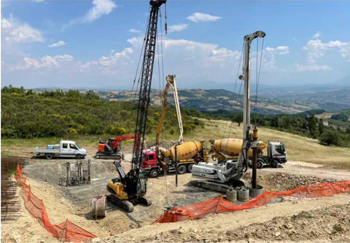
Figure 11-1 - Works on site for WTG 08
