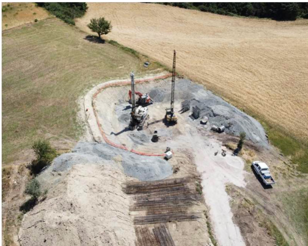
Figure 11-5 - Works on site for WTG 09
