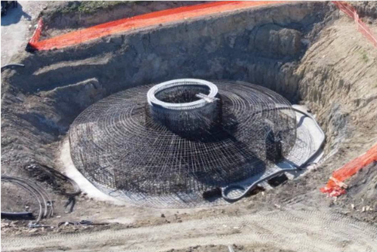
Figure 11-1 - Works on site for WTG 08
