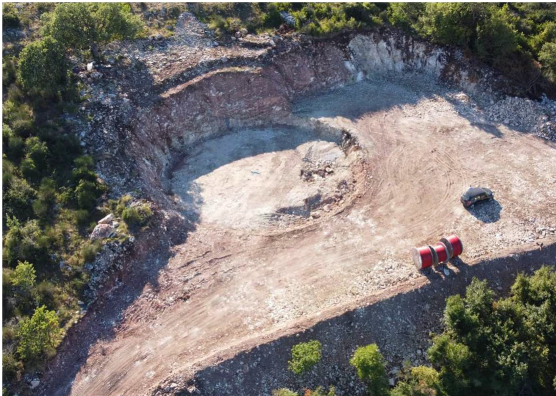
Figure 11-5 - road and crane pad preparation for WTG 18
