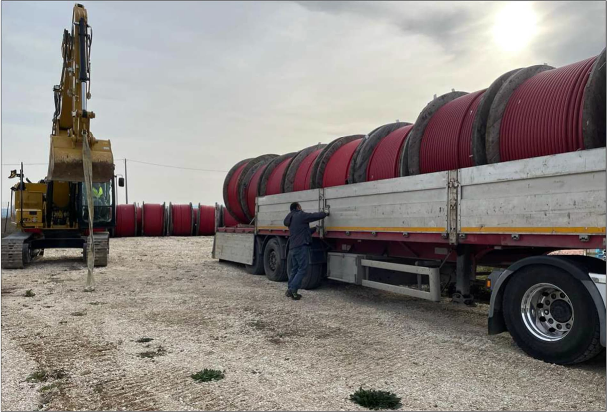
Figure 11-7 - MV cables unloading at site
