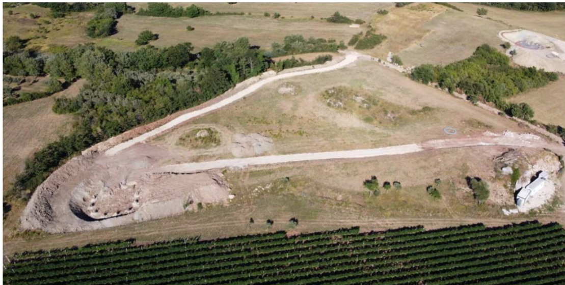
Figure 11-3 - Works on site for WTG 10
