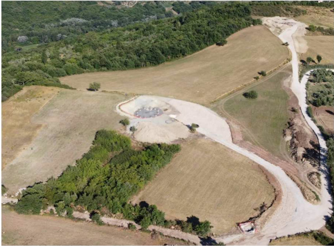
Figure 11-2 - Works on site for WTG 09
