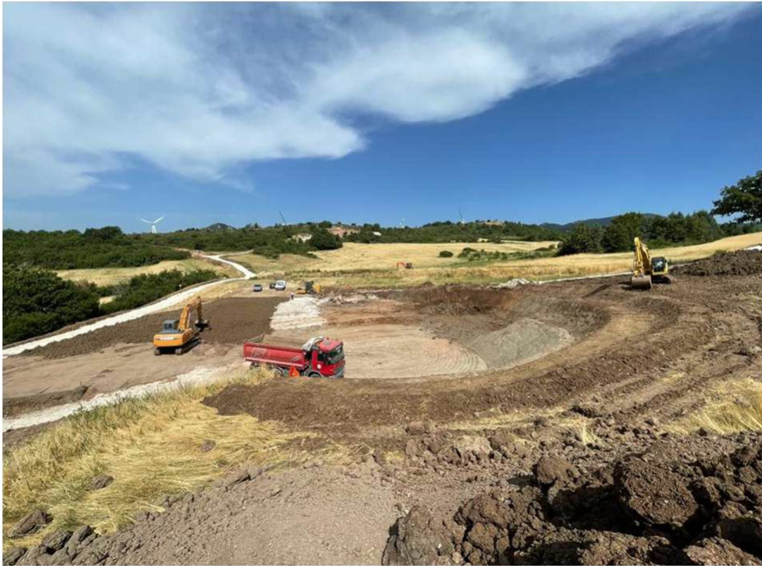
Figure 11-4 - Works on site for WTG 11
