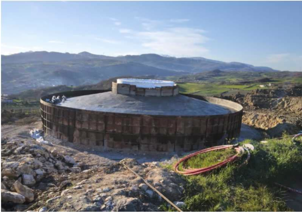
Figure 11-3 - WTG G03 foundation poured
