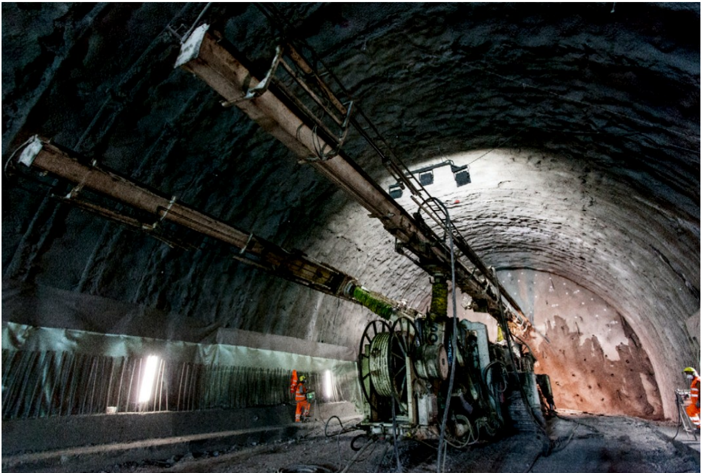
The Soilmec drill rig is being used to install the 40 - 90 rods used to re-inforce the conventional tunnel
