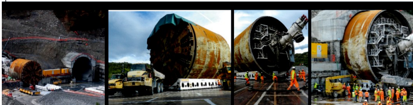
Photographic sequence showing the removal, turning, and repositioning of the 15.6m diameter TBM for the second tube
