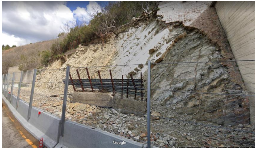
Figure 5-2 - Landslide on SS 90
