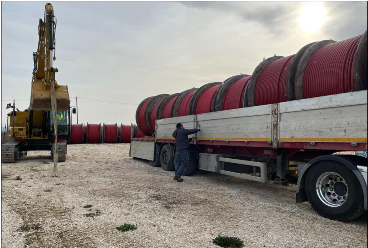
Figure 11-3 - MV cable unloading at site
