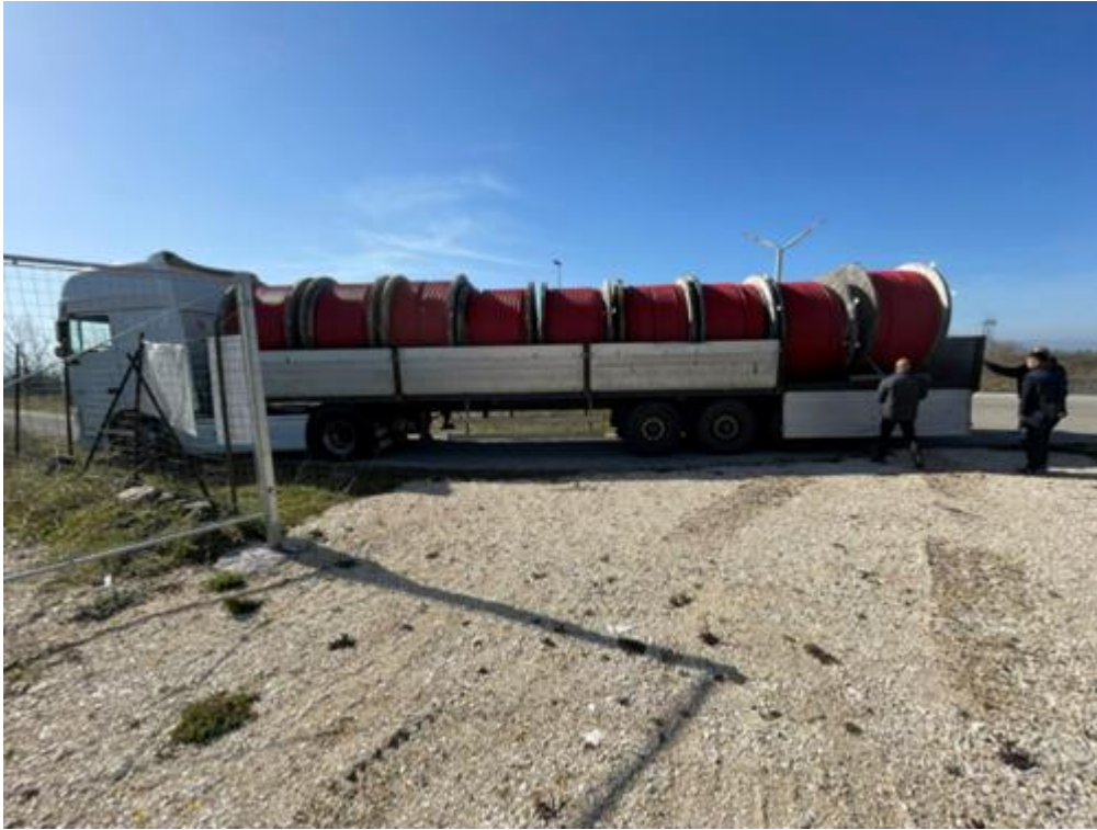
Figure 11-2 - Start of MV Cable delivery activities at site
