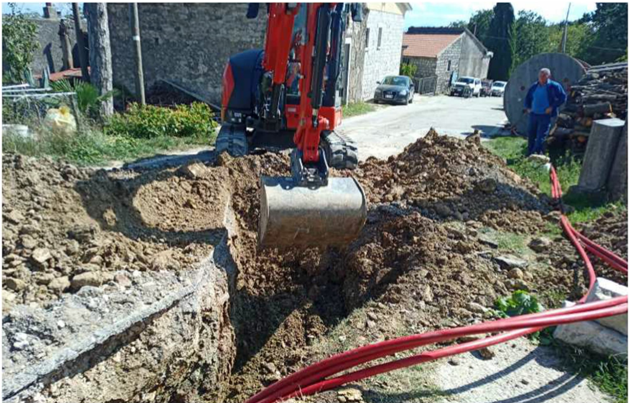
Figure 11-4 - MT cable works
