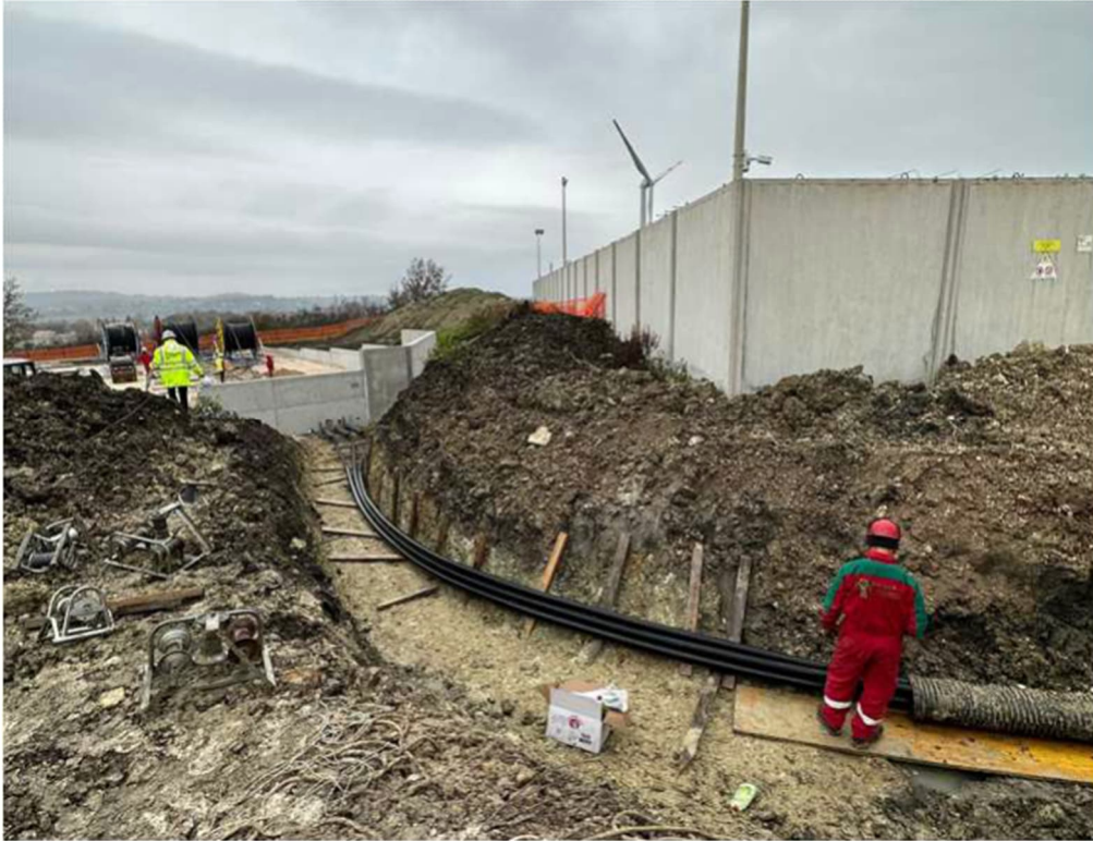
Figure 11-1 - HV cables laying
