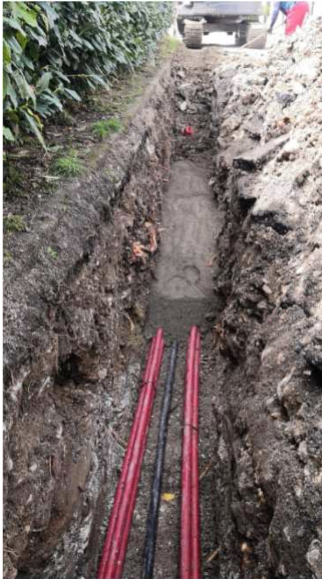
Figure 11-3 - MV Cable duct works
