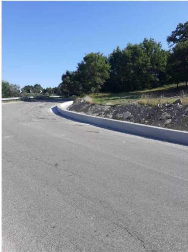
Figure 11-3 - Restoration work on external roads ongoing
