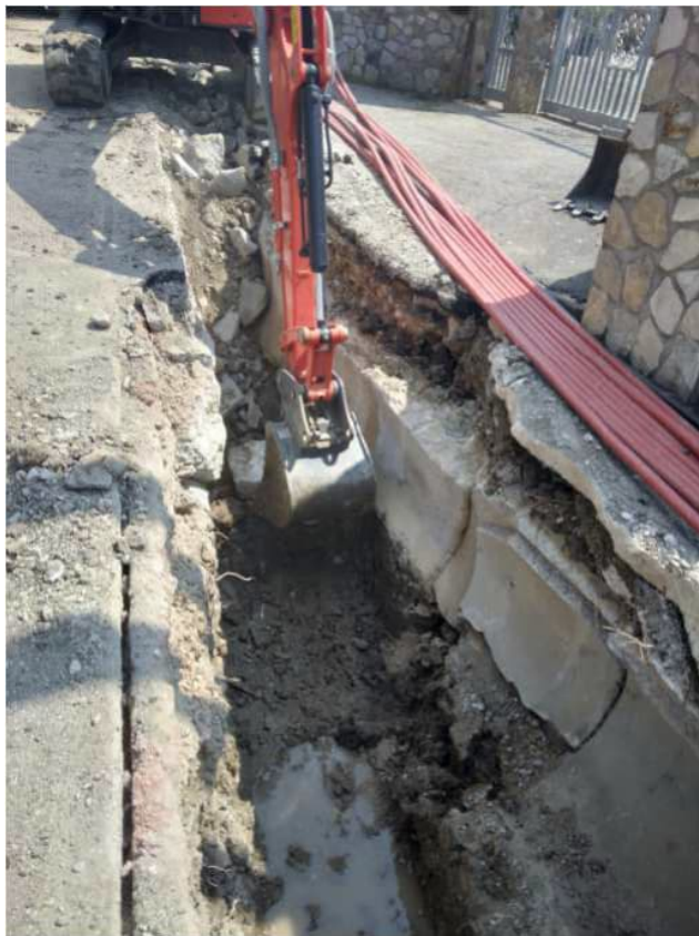
Figure 11-4 - Laying of MV cables on external roads
