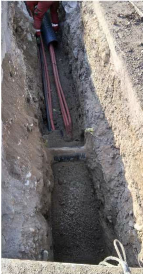
Figure 11-2 - MV cable duct works ongoing
