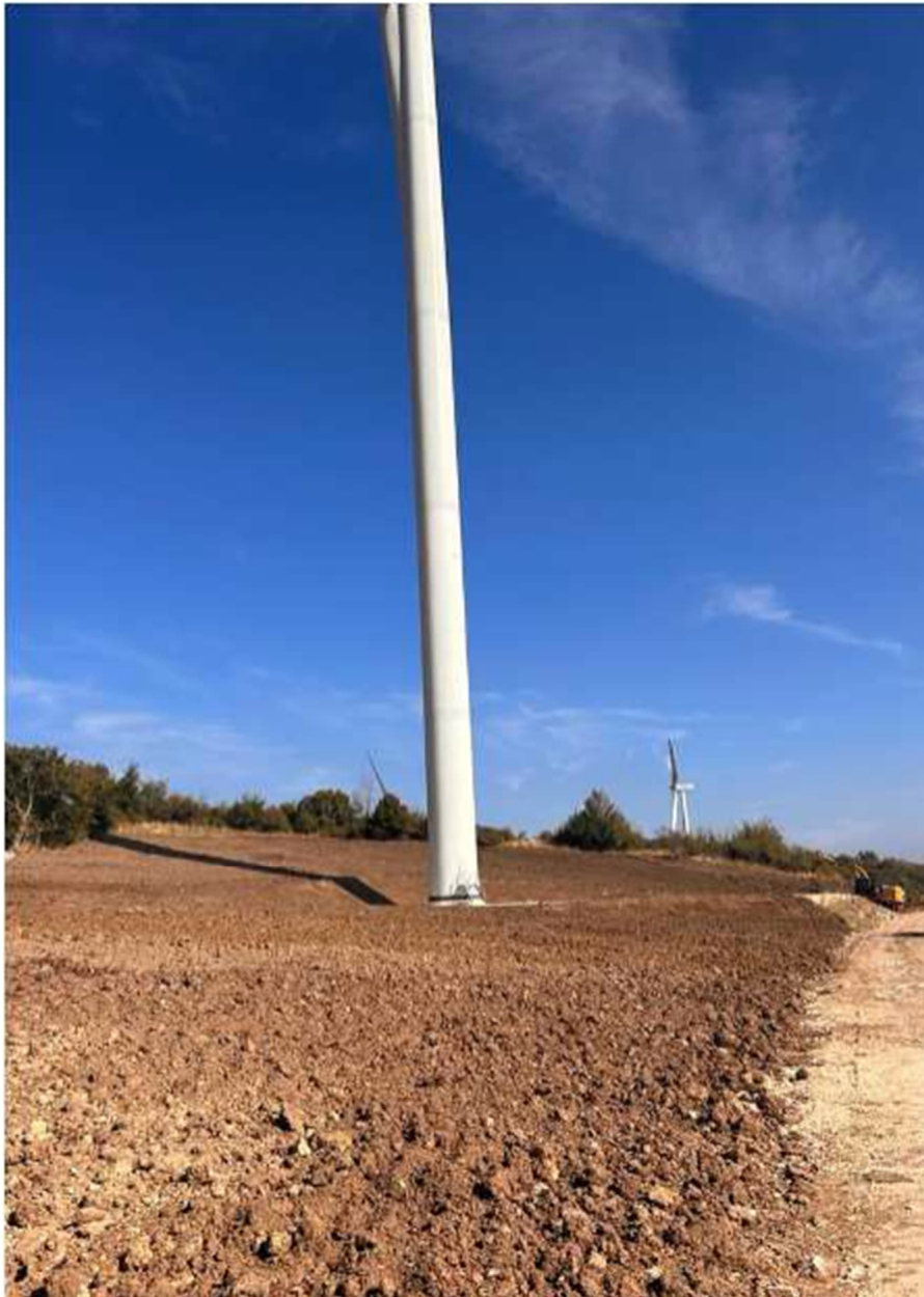
Figure 11-1 - Restoration works on pads ongoing
